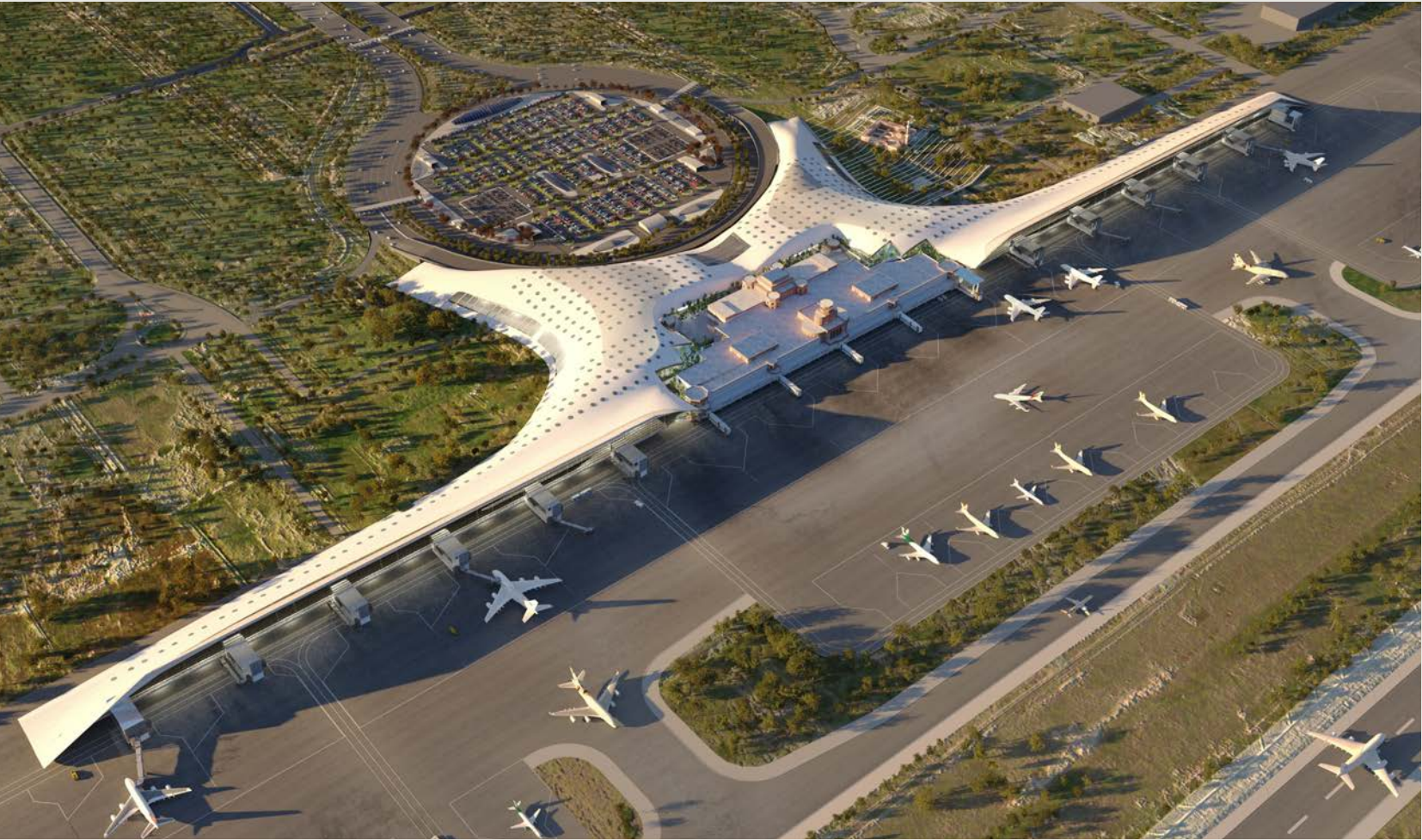
Development of Projects for EPC Contractors
